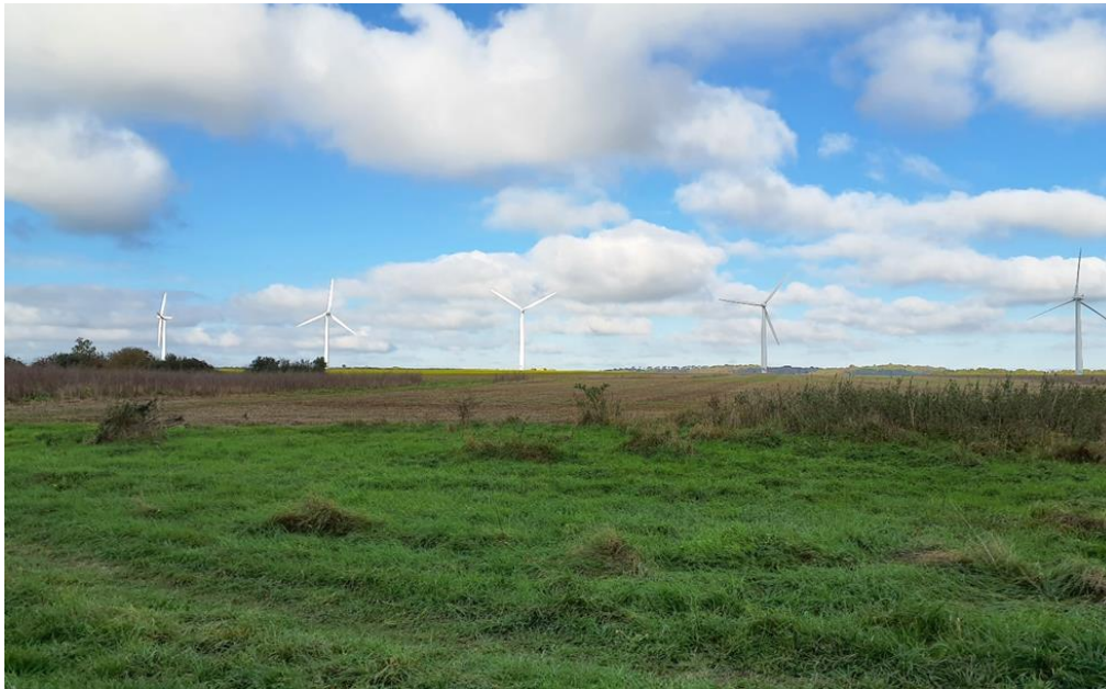
Figure A.24: Westmill Wind Farm near Watchfield
