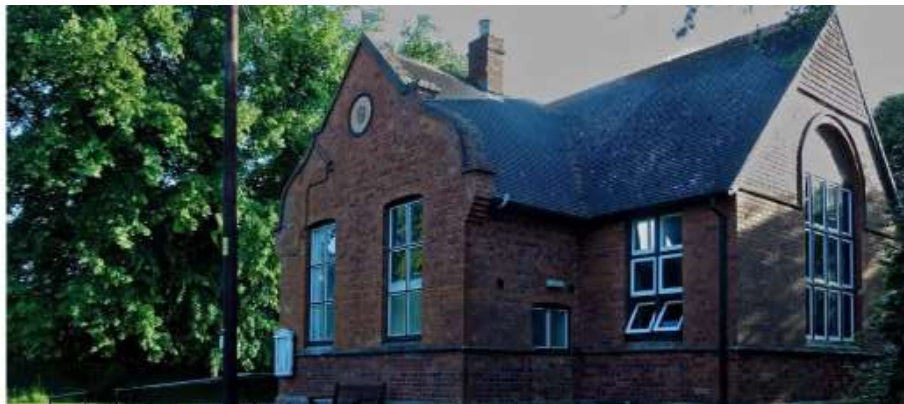
Fig.10: Pyrton village hall
