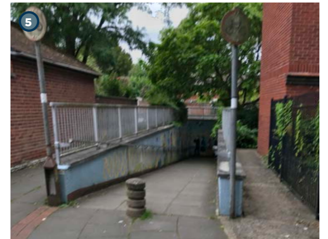
Fig 5.7: View of the pedestrian subway under Stratton Way, linking the north of Abingdon with the town centre
