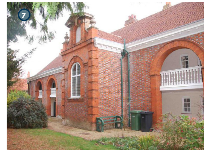
Fig 4.29: View of Grade I listed Brick Alley Almshouse built in c. 1718
