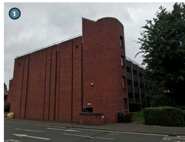
Fig 5.3: View of The Charter Car park from Broad Street
