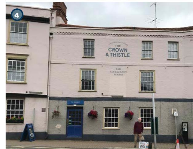
Fig 4.26: View of The Crown and Thistle Hotel and Public House on Bridge Street, a Grade II listed building originally built in c. 1605
