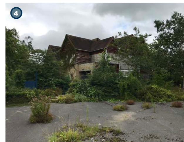
Fig 5.24: View of the southern part of the Upper Reaches building
