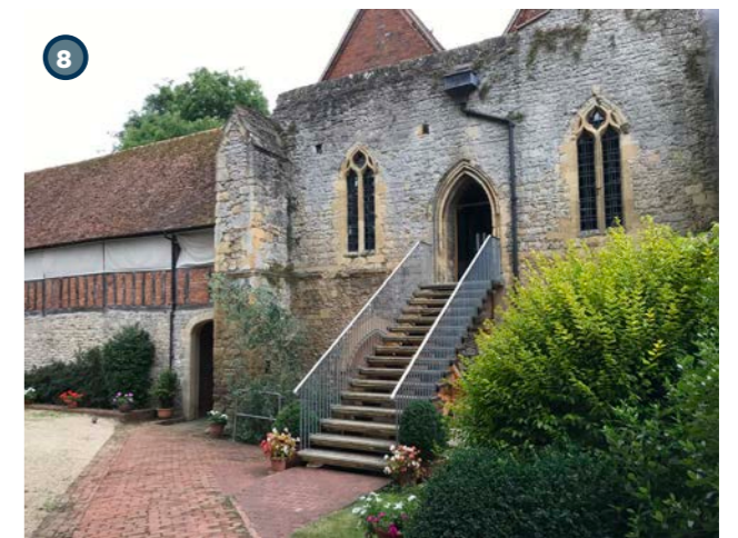
Fig 4.19: View of Abbey Checker, adjacent to the Unicorn Theatre and the Long Gallery
