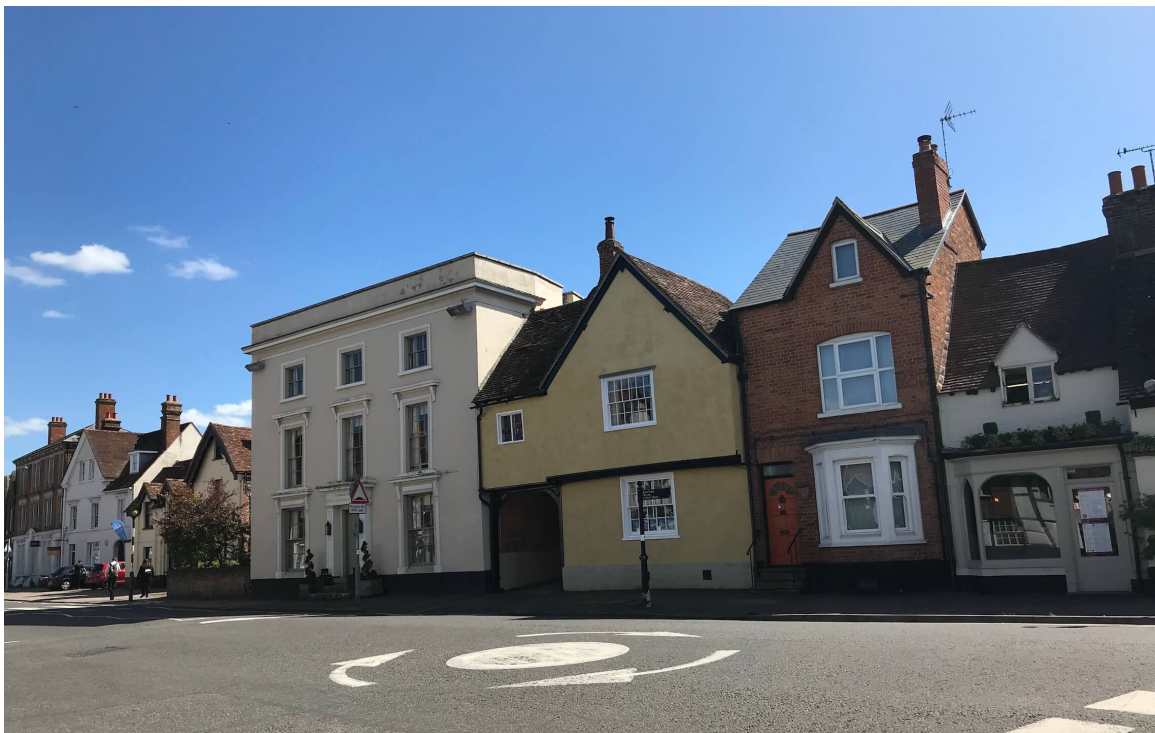
Figure 22: Buildings in the 'Historic Core'
