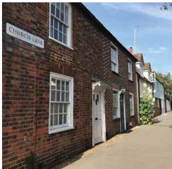
C18 vitrified header brickwork, Church Lane
