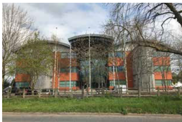
Former Habitat showroom and warehouse
