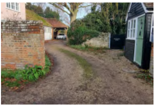
Poorly finished surface treatment and impacts from tree roots are problematic
