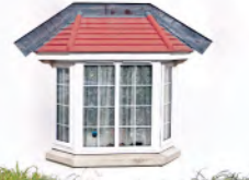
Preformed bay window canopies in GRP with poorly coloured roofing and excessive use of flashing is not in keeping with the character of the area
