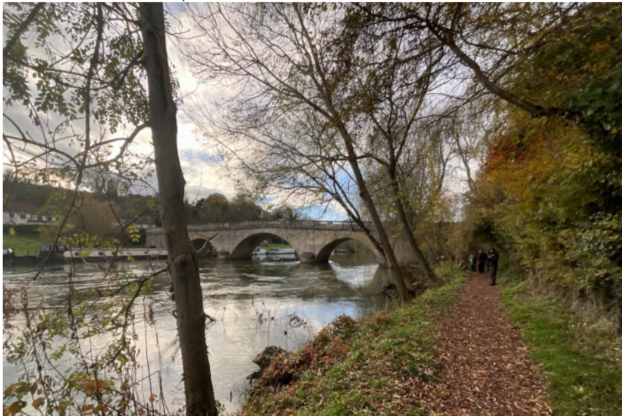
The Grade II* listed bridge with its graduated segmental arches, built of Limestone ashlar and some red brick - built in 1826-7
