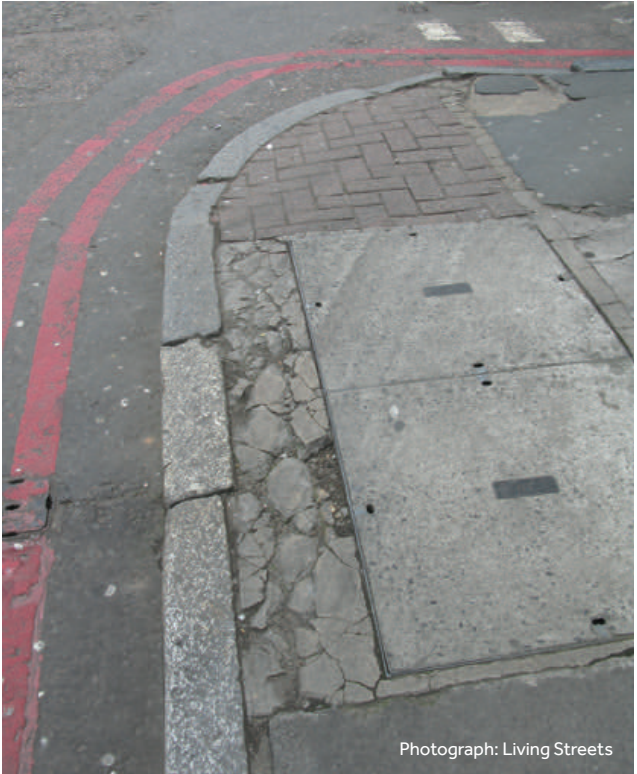
Poor quality pavement
