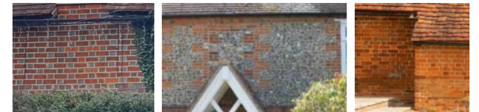
Flemish bond with contrasting headers
