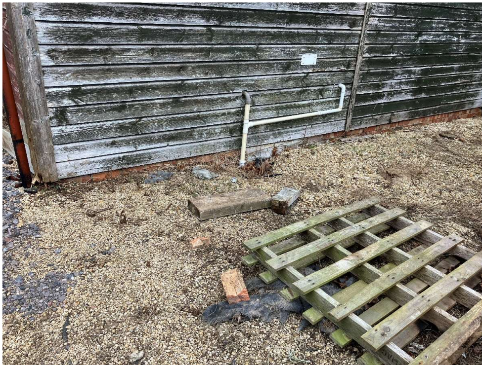
Exposed brick plinth wall to base of southern end gable
