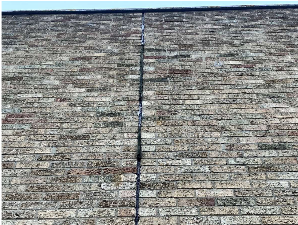
Northern end wall to sports hall with missing joint sealant and filler projecting out from movement joint
