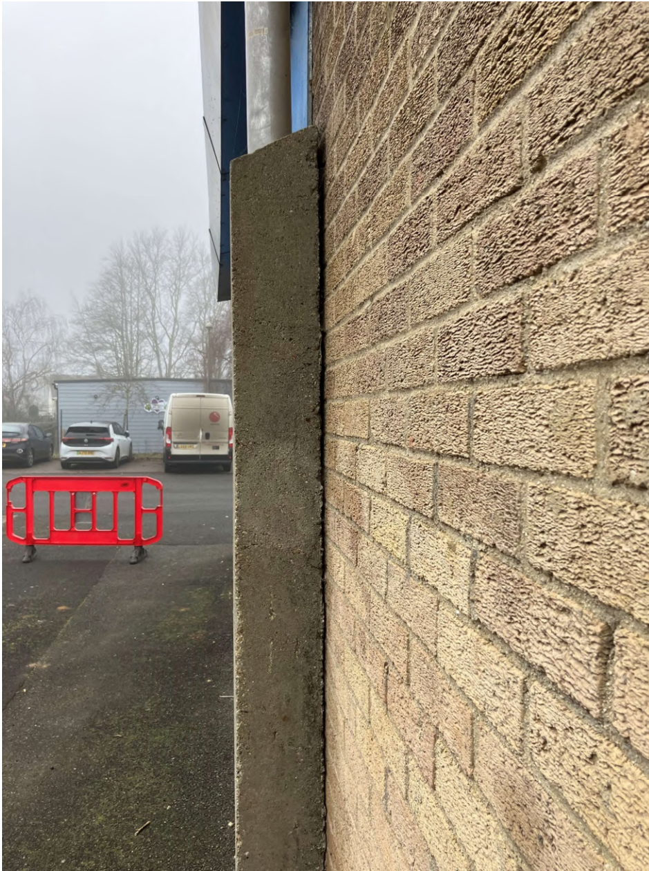
Concrete encasement to rainwater down pipe coming away from external masonry wall
