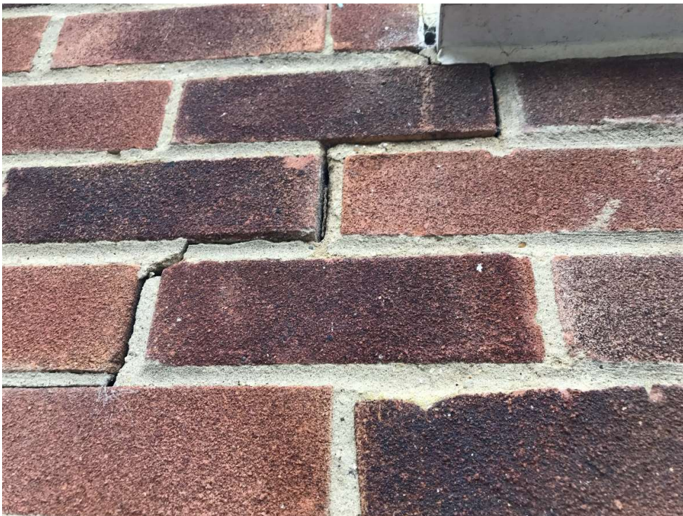
Cracking to external (East) elevation of Building B
