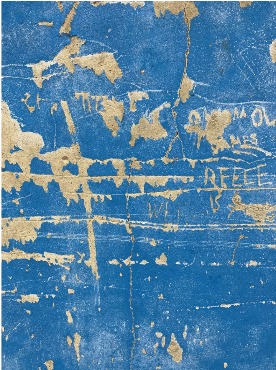
Near vertical; crack to side wall of foyer
