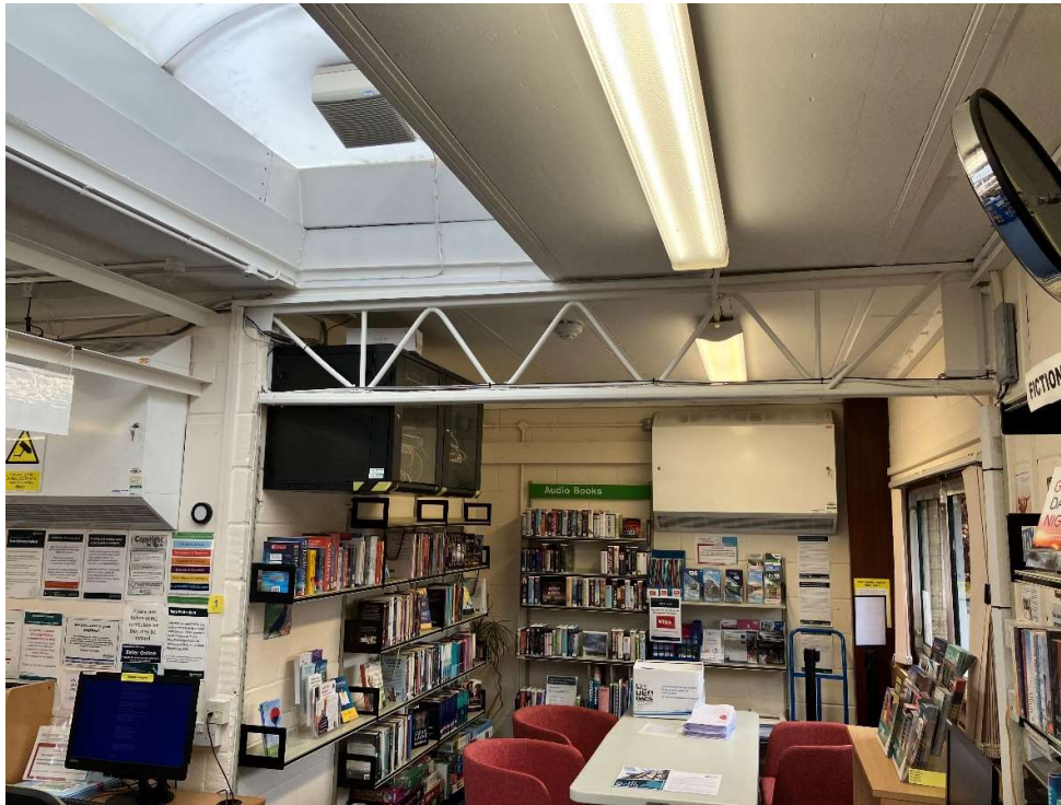
Short span roof truss to south-east corner of building
