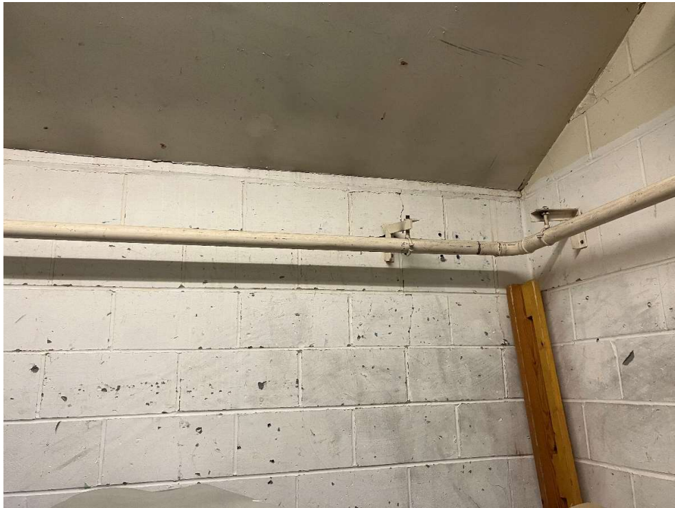
Minor crack to internal blockwork wall at services support location in lean to store at south end of sports hall
