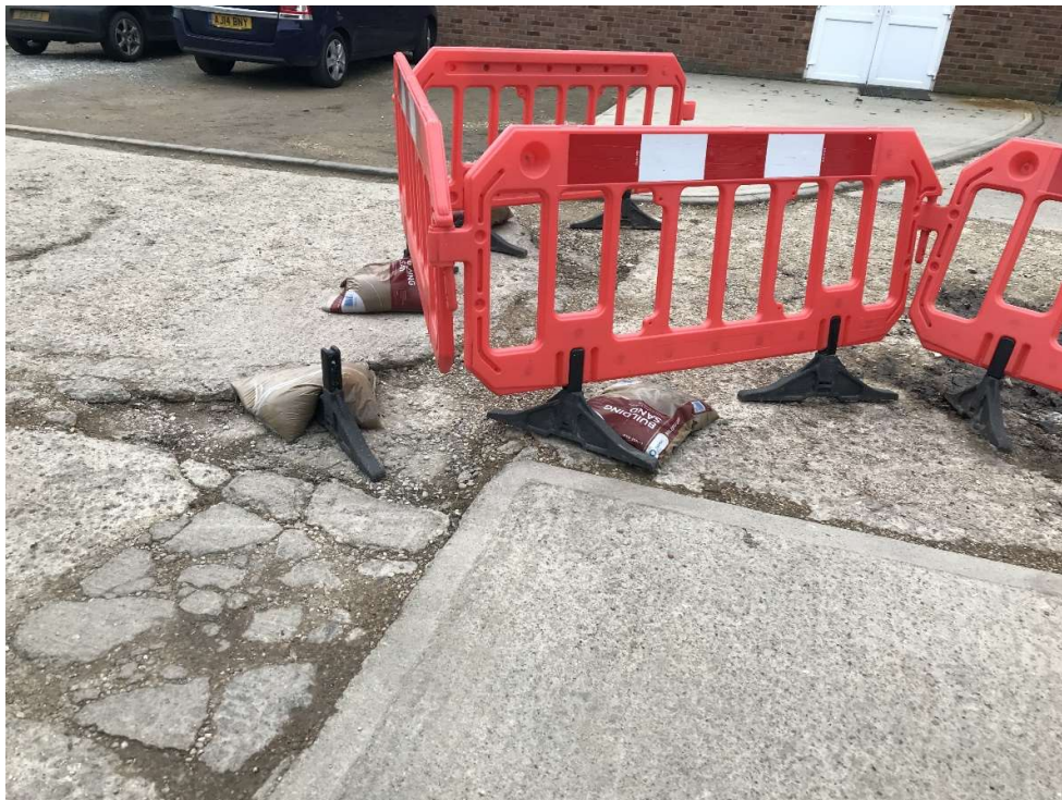
Concrete hard standing showing areas of significant degradation.
