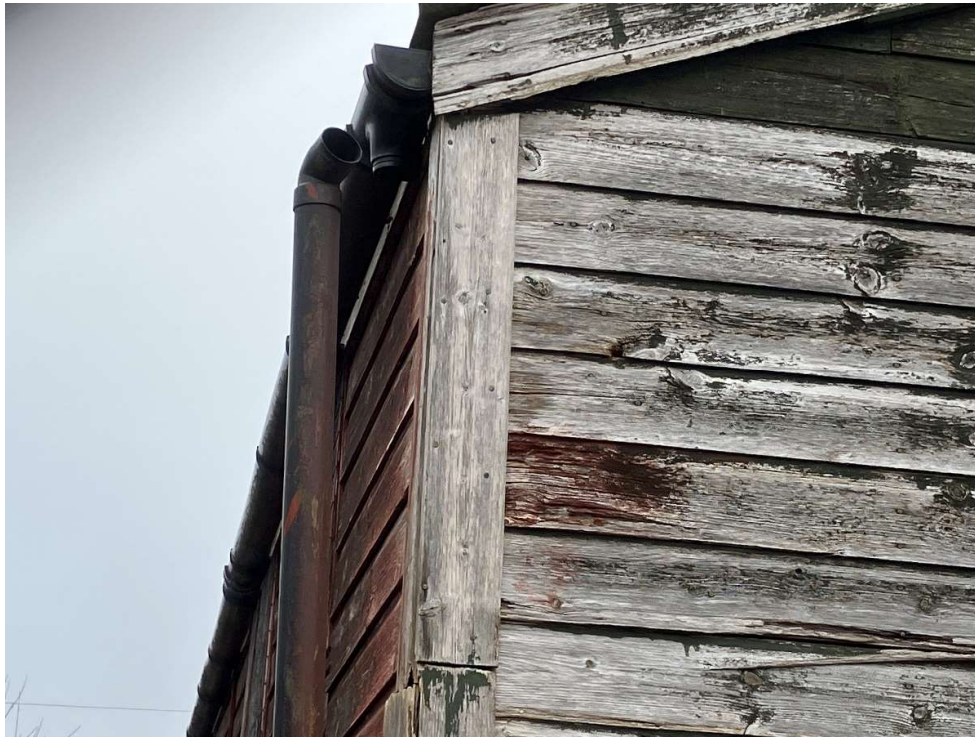
Disconnected rainwater downpipe to south west corner
