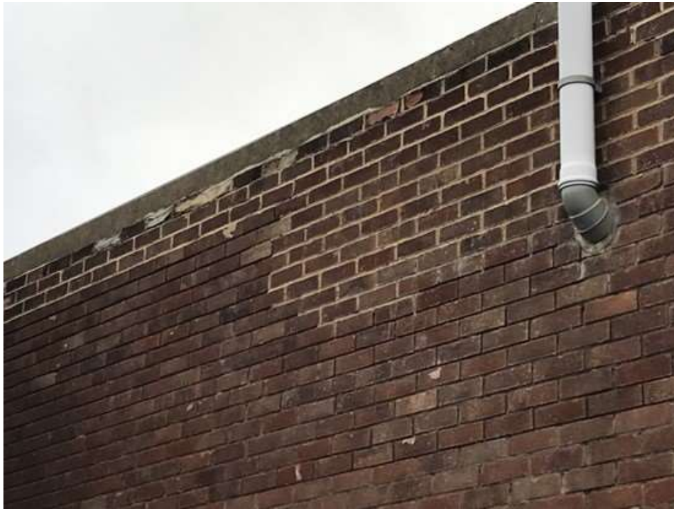
External masonry elevation with repairs to masonry evident and spalling of brickwork
