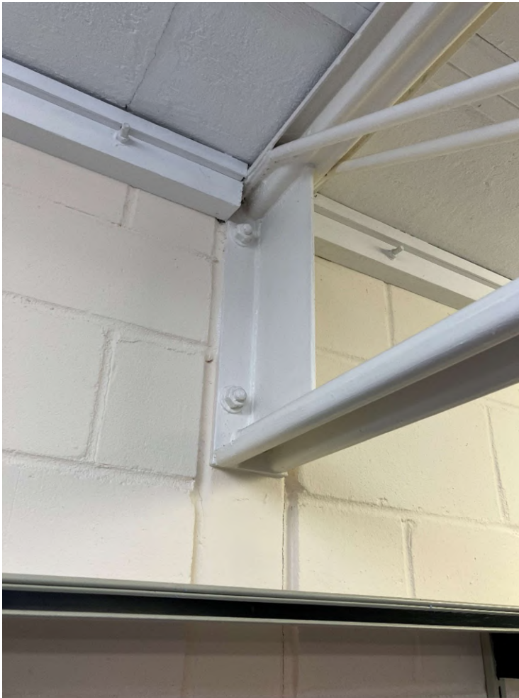
Truss end to steel column connection
