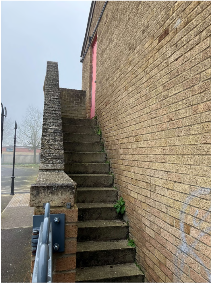
External fire escape from mezzanine floor
