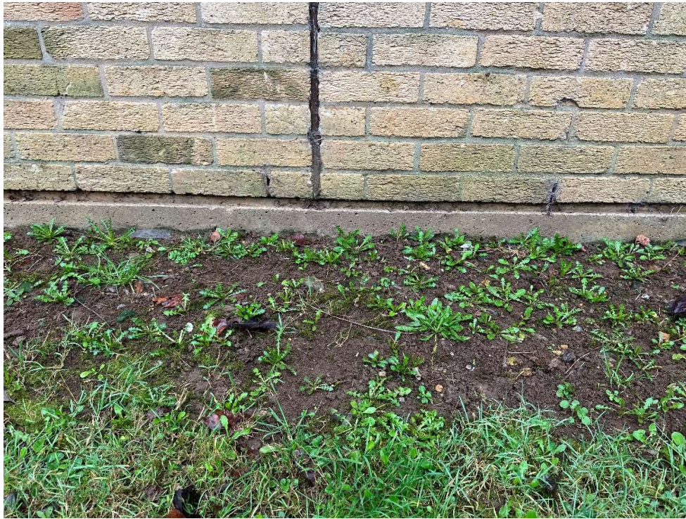
Possible edge of sports hall floor slab supporting external wall
