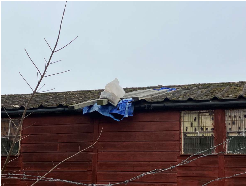
Apparent roof repair to eastern roof slope
