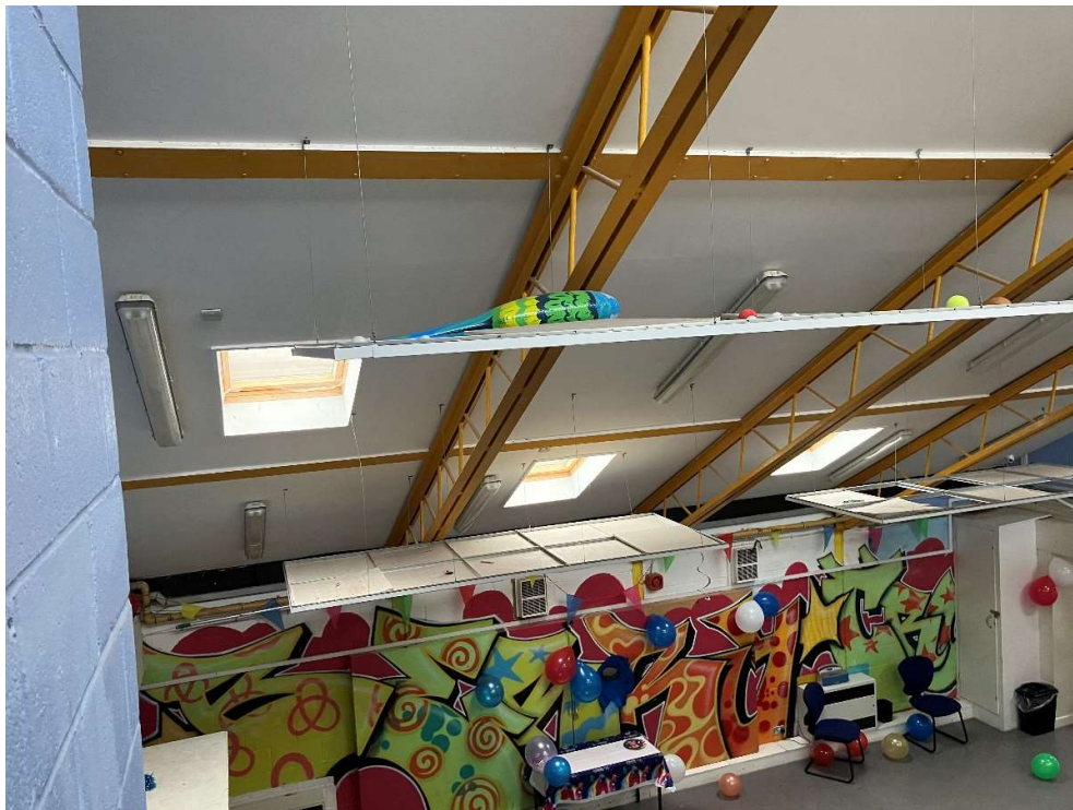
Exposed roof trusses from mezzanine
