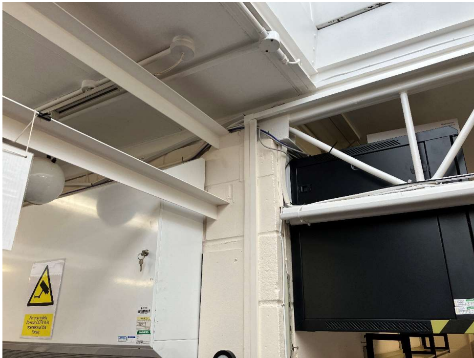
Internal loadbearing wall support for short span roof truss
