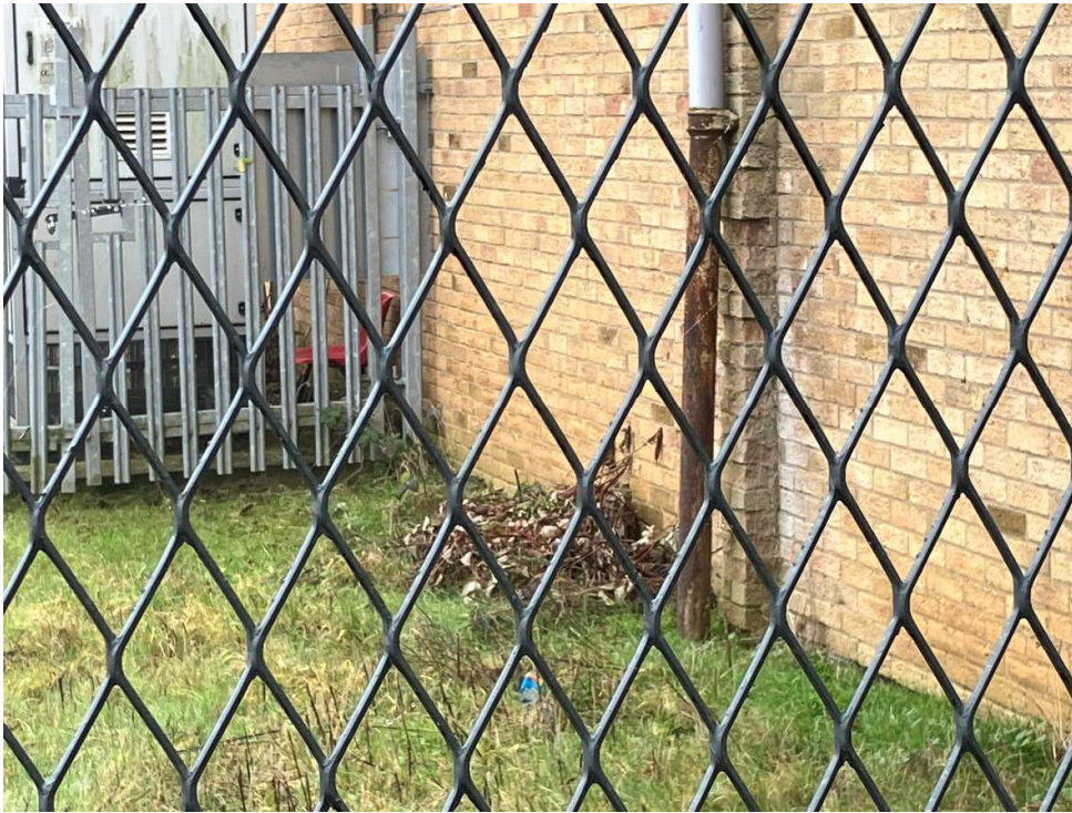
Spalled brickwork and removed concrete encasement to rainwater down pipe on eastern elevation
