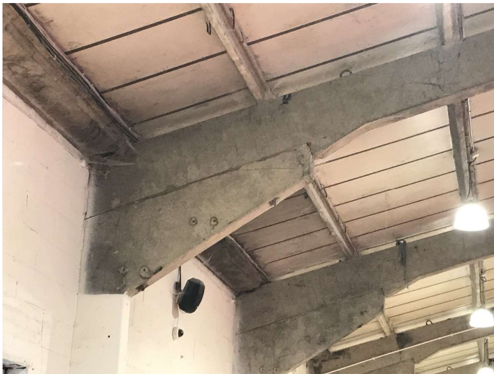
Precast concrete rafters, columns and haunches with purlins visible over the top of the rafter.
