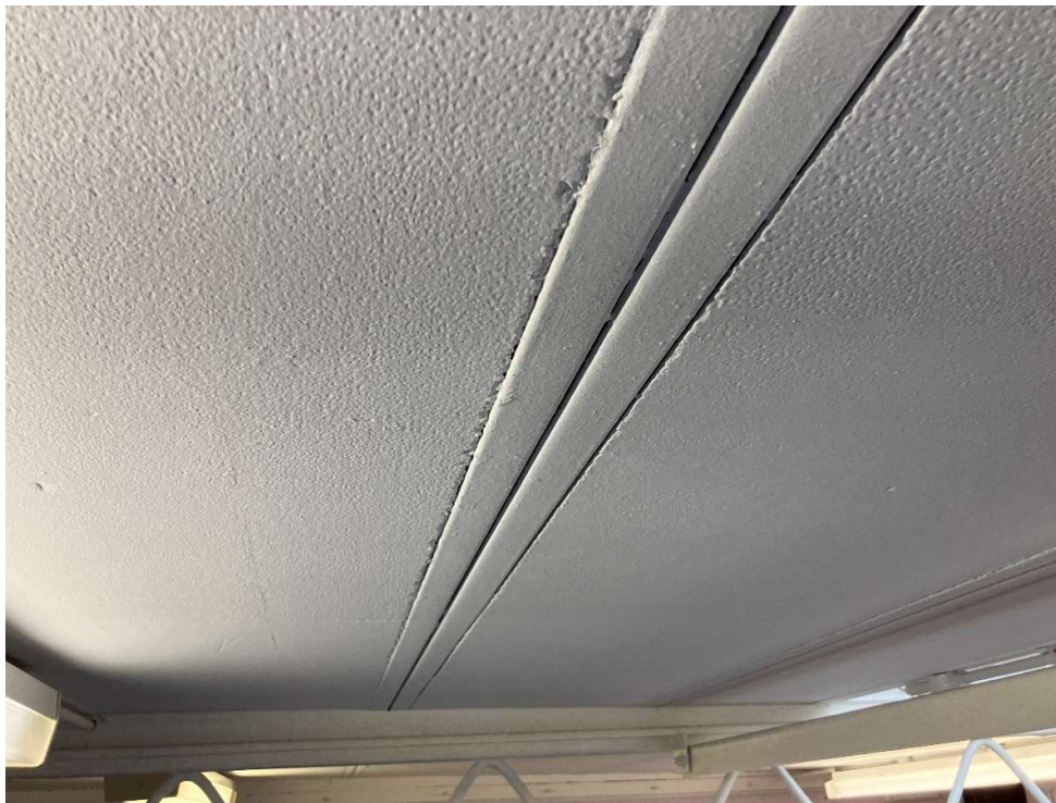
Joint of painted galvanised steel channels between adjacent roof panels
