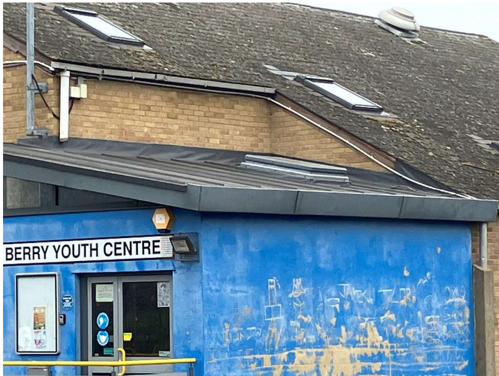
Standing seam roof to entrance foyer
