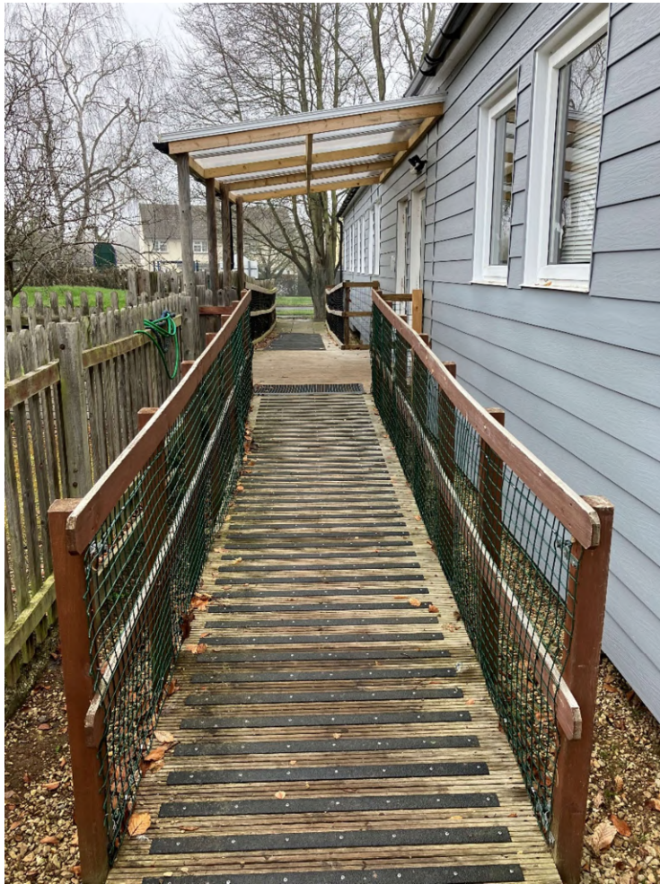
Timber access ramp and covered porch to southern elevation
