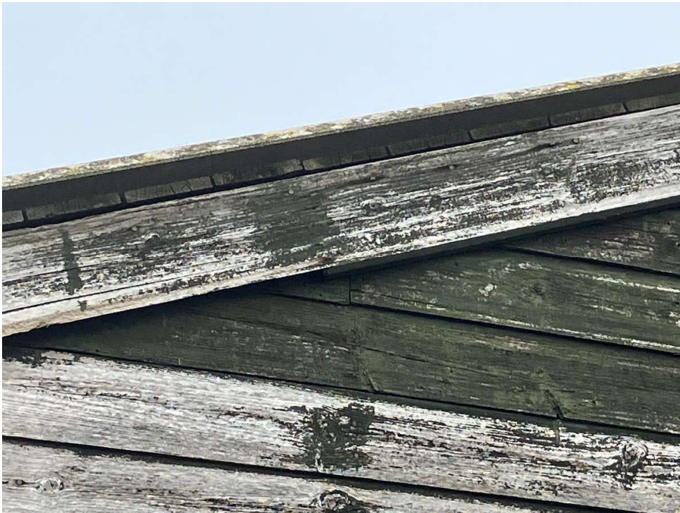
Exposed ends of roof boarding beneath asbestos roof sheets
