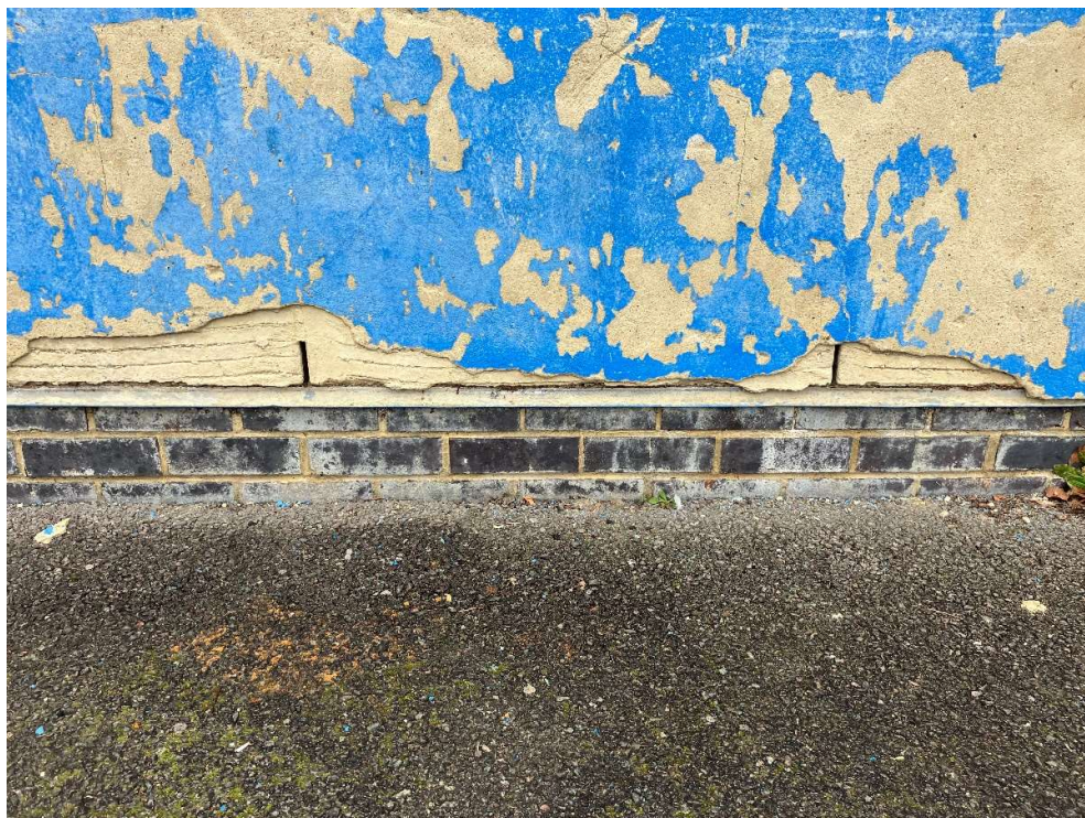
Missing cavity vents to side wall of entrance foyer
