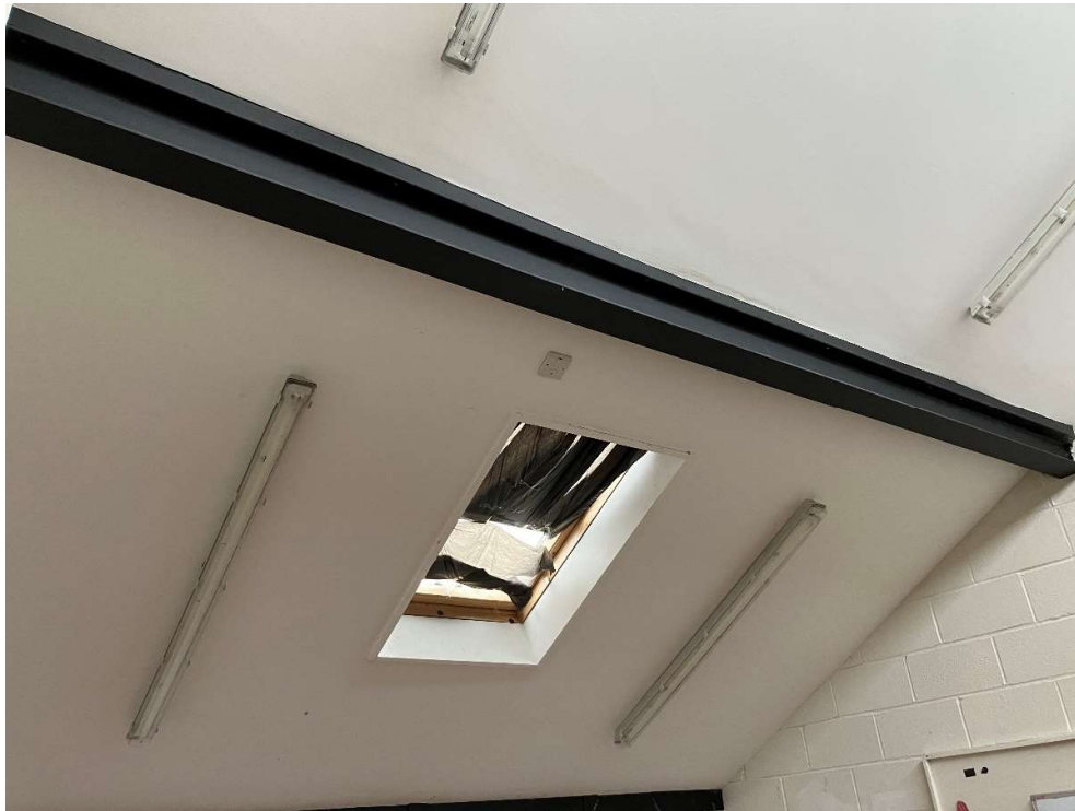
Exposed roof support beam in mezzanine meeting room
