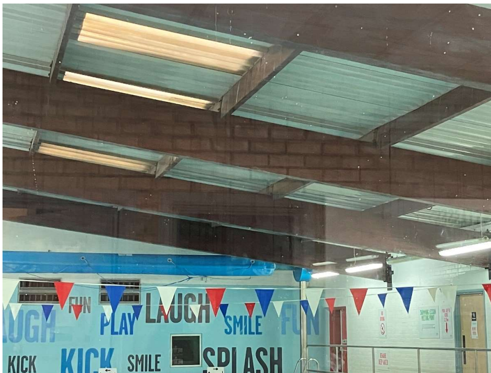
Glulam timber roof over swimming pool
