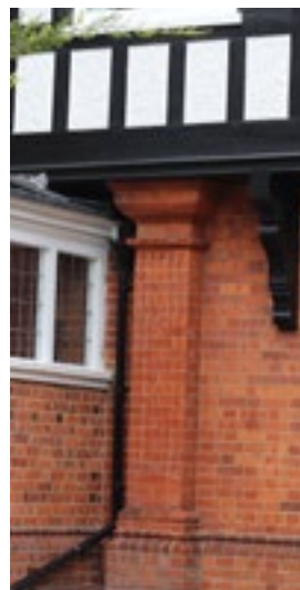
Fig 75. Brick pilaster
