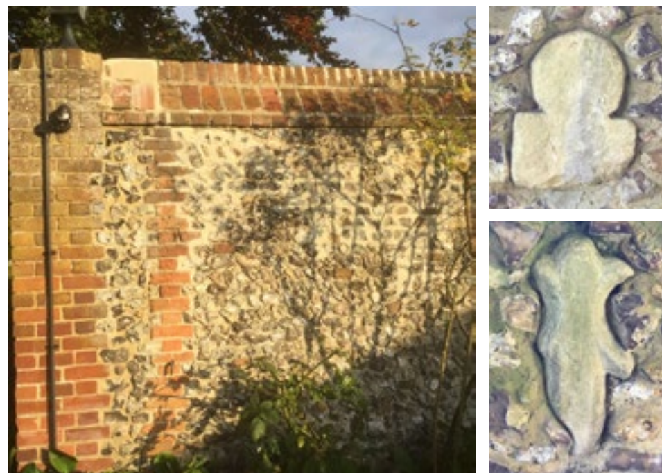
Fig 50. Churchyard wall, flint and brick, and worked stones
