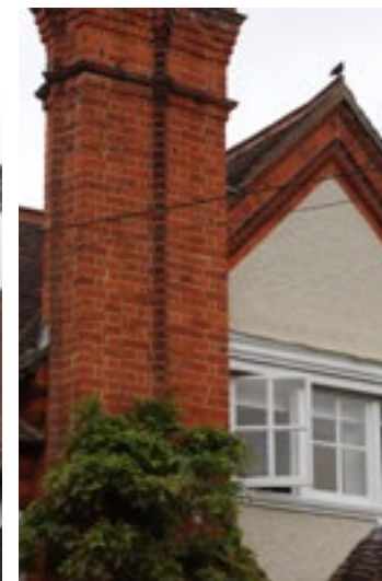
Fig 77. Brick moulding
