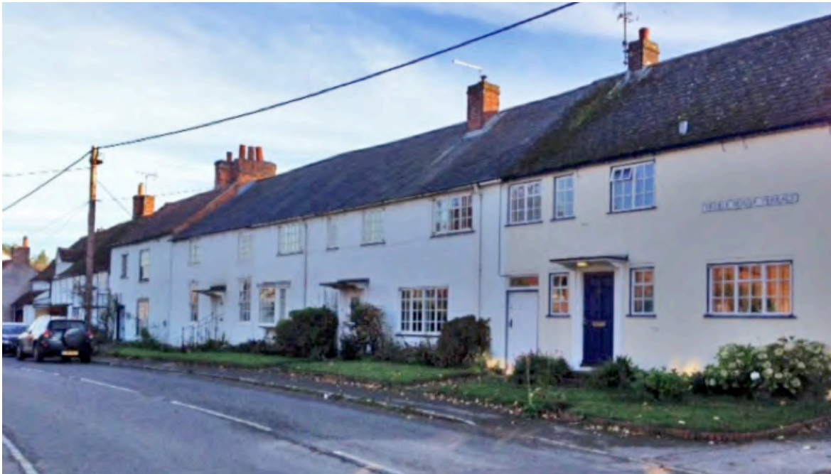
Fig. 20: Former commercial property at Treble House Terrace, London Road
