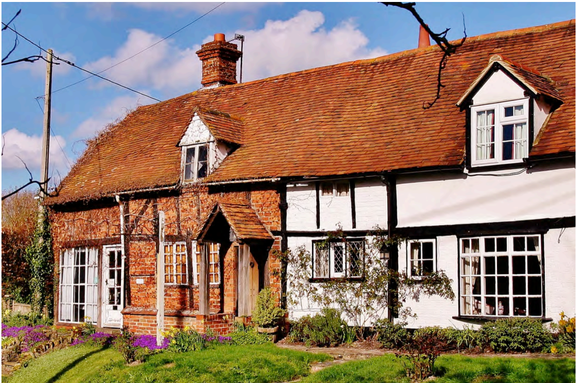
Fig. 25: Lantern Cottage, on left, showing evidence of former tea shop.
