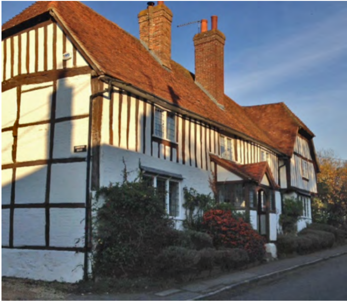
Fig. 22: Corrydon House, London Road showing the higher-status close studding on the front elevation with small square panelling to the side elevation
