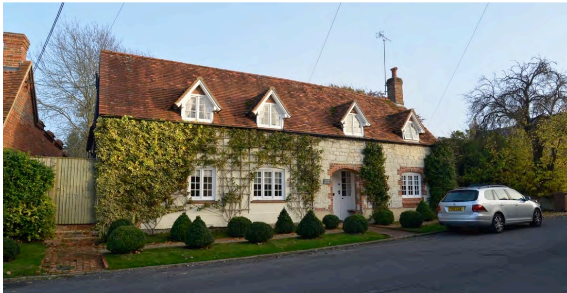
Fig. 24: Manor Cottage, constructed of chalk block or clunch
